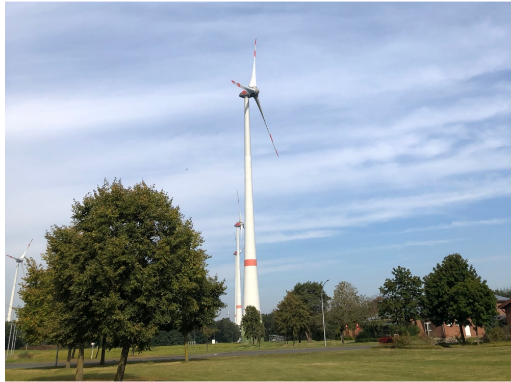
Turbines at Saerbeck's Bioenergie Park.
